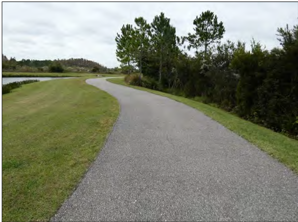
Enclave Asphalt Path
