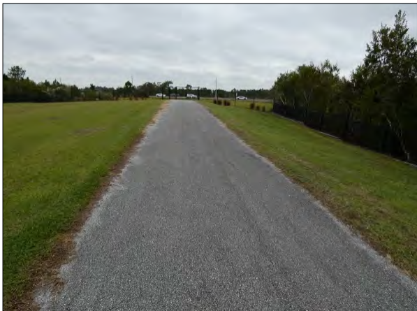
Windsor Asphalt Path
